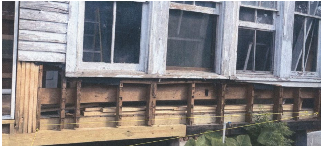
South (Rear) Before Work
