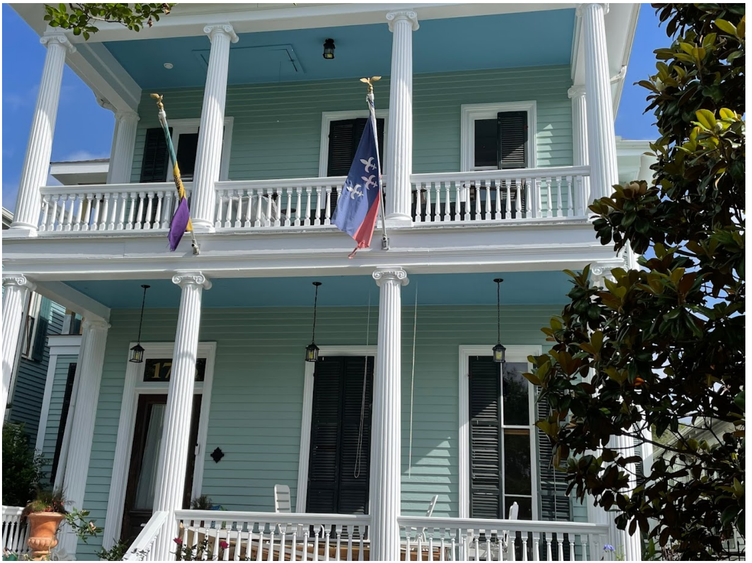
Front porch trim before rot
