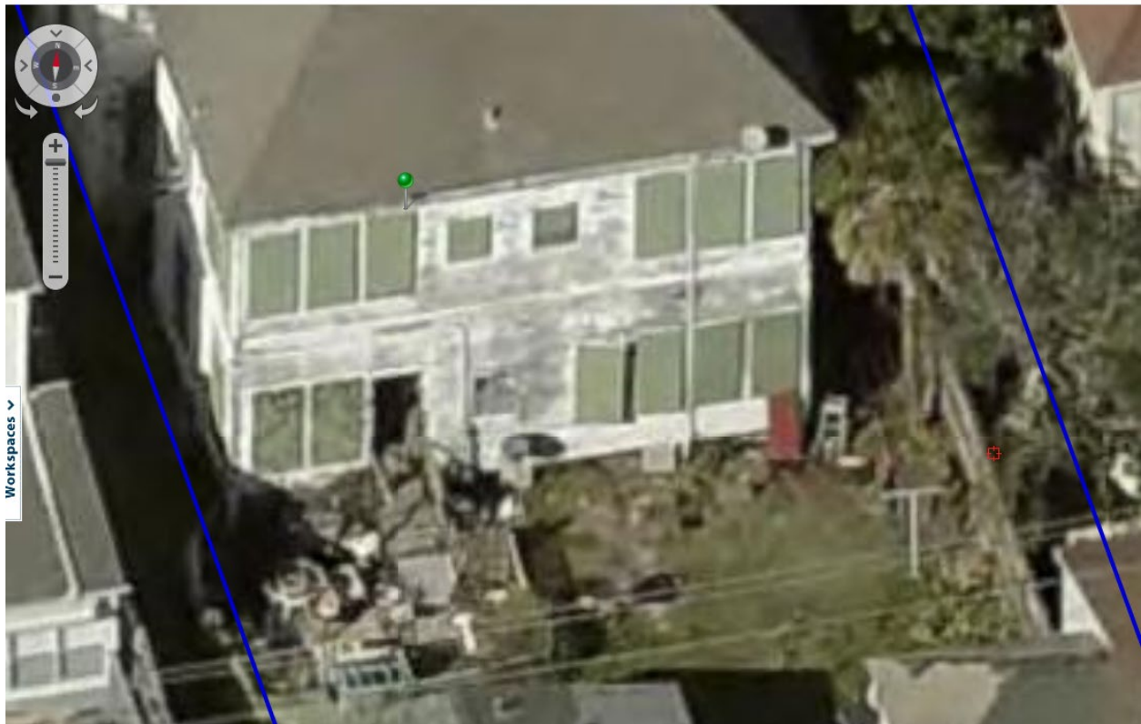
South (Rear) Before Work
