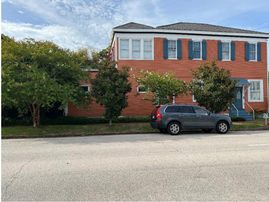
South Elevation, 1202 & 1208 Postoffice, August 2022
