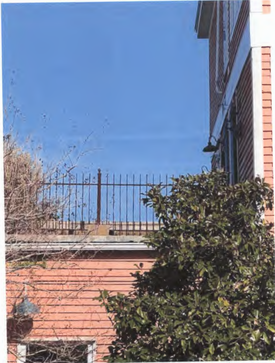
South side, Postoffice Street view, steel railing existing
