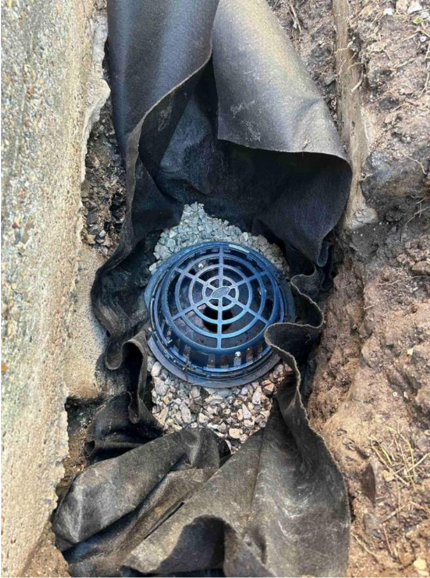
Drain Frame and Grate, Aggregate, Geotextile
