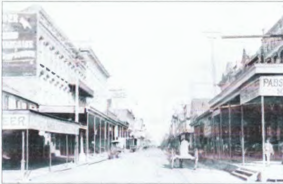
Taken in 1894 of Market Street, looking east from Twenty-fifth Street, this photograph shows the R. F. Martin and Company (1878) and Lalor (1894) Buildings, which are located along the right of the photograph. Without awnings, the flavor of the street is completely different. The two larger buildings on the left-side of the photograph have been demolished.
