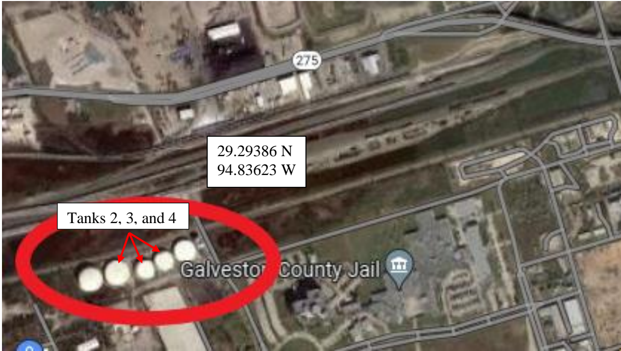
Figure 1: Latitude/Longitude of Site and Tank Identification
